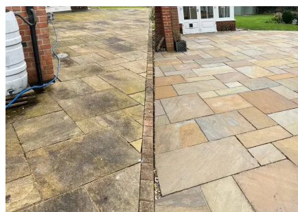
Sandstone patio — before and after.
